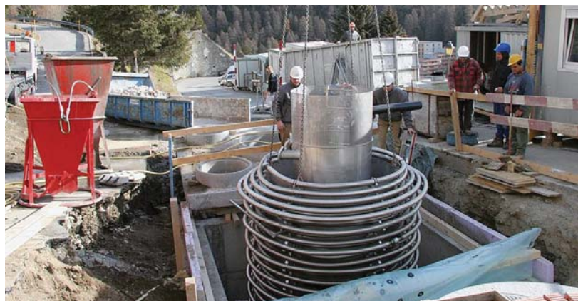
This waste water shaft is used as a primary source for DHW heating.
