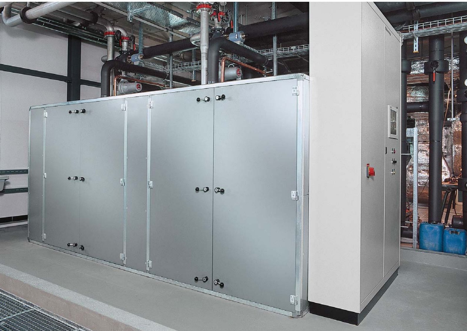
Water/water heat pump with a heating output of 500 kW
