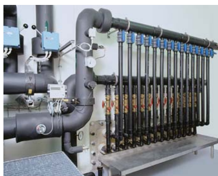
Geothermal probe manifold
