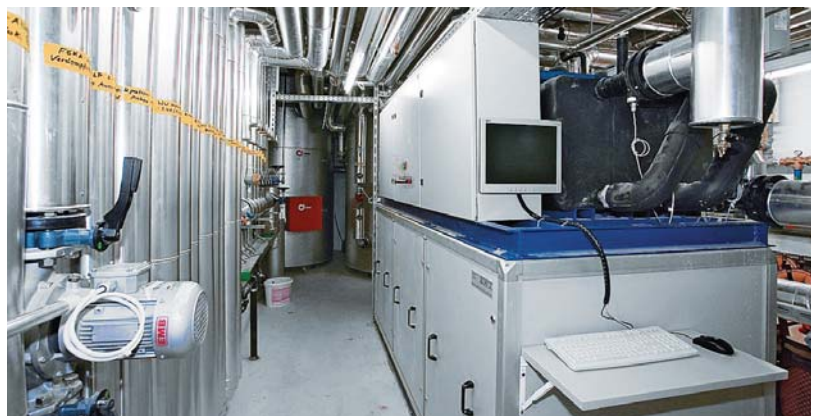
A waste water heat pump with 150 kW output for DHW heating
