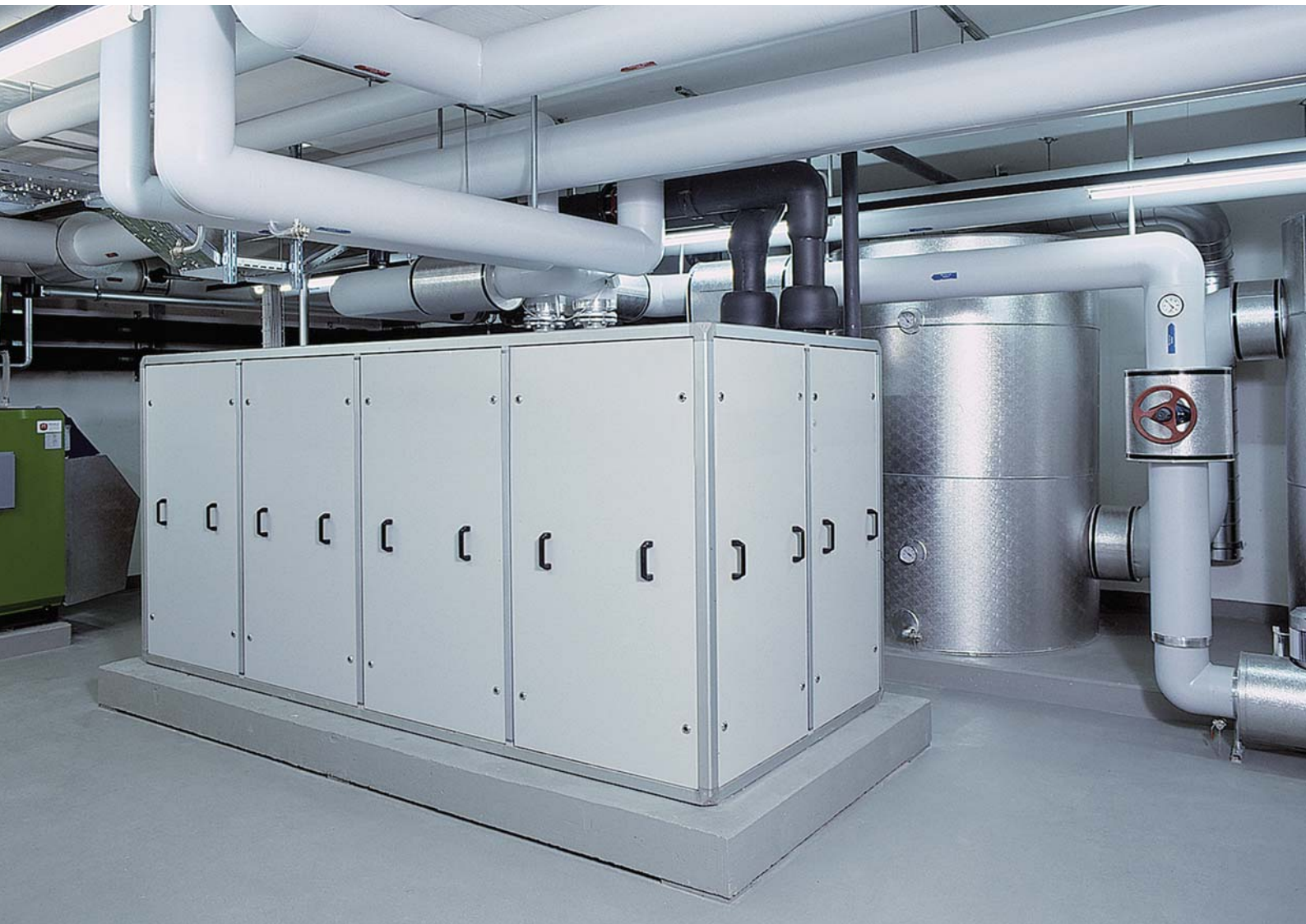
Brine/water heat pump with a heating output of 290 kW
