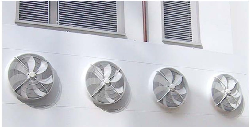
Glycol dry coolers for air/water heat pumps, mounted on a wall
