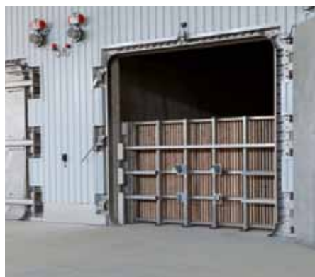
Digester gate with substrate barrier
